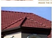
ROOF WORK • MANGALORE TILES FOR ROOFING GIVES THE STRUCTURE TOTALLY DIFFERENT ELEGANCE BY ITS BEAUTY. • THEY GIVE US FEEL OF TRADITIONAL INDIAN HOMES. • TILES DON'T ABSORB MUCH HEAT FOR SUN, THEY HELP MAINTAIN PLEASANT INDOOR TEMPERATURE.
